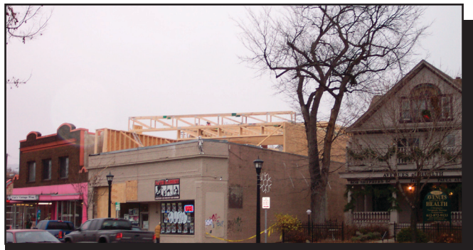
Beginning framing of second story addition
