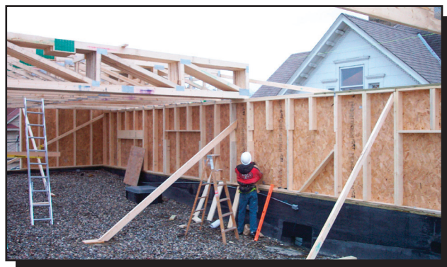
Trusses added and view of inside with old roof
