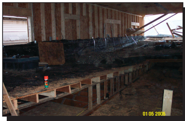
New floor being installed and old roof being removed
